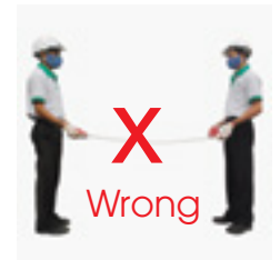
The board is sagged when being carried horizontally.
