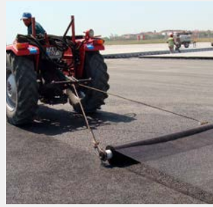
Installation of ADFORS GlasGrid at Atatürk Airport, 2010
