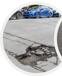
Example of cracking for local repairs
