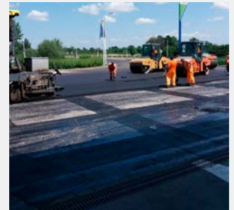
Installation of ADFORS GlasGrid in Belgrade, 2018
