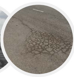
Example of cracking for area-wide repairs
