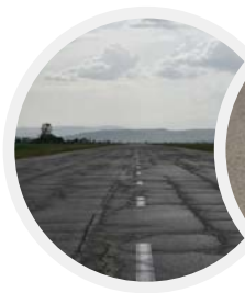
Example of cracking for area-wide repairs
