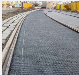
Installation of ADFORS GlasGrid in Prague, 2013
