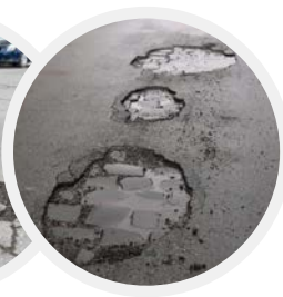
Example of cracking for local repairs
